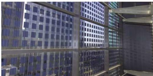
THE "HERON TOWER" IN LONDON WITH THE SEMI-TRANSPARENT DOBLE SKIN - BIPV FAÇADE (PICTURE: P. BONOMO).
