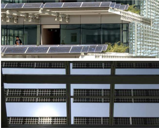
PV SHADINGS IN THE SIEEB BUILDING, BEIJING, MARIO CUCINELLA ARCHITECTS (SOURCE: WWW.SINOITAENVIRONMENT.ORG/ )
