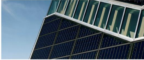
WARM FAÇADE BIPV SOLUTION, MONTE ROSA HUT (ZERMATT, SWITZERLAND) (ARCHITECT: ETH STUDIO MONTE ROSA)
