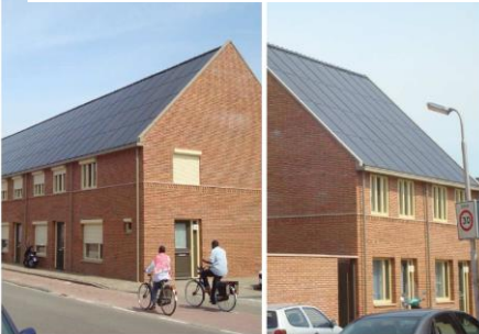
SCX SOLOROOF AS BIPV FULL ROOF SOLUTION (TILBURG, THE NETHERLANDS), 75 TERRACED DWELLINGS
