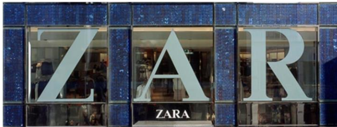
Fig. 3.B.24: warm façade solution. Zara Fashion Store, Cologne, Germany, Architekturbüro Angela und Georg Feinhals: opaque monocrystalline cells combined with transparent glazing in post-beam curtain wall structure, © Solon.
