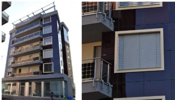
WARM FAÇADE BIPV SOLUTION, PALAZZO POSITIVO (CHIASO, SWITZERLAND) (ARCHITECT: TOUR BAUMANAGEMENT AG, BAD RAGAZ, PICTURES: F. FRONTINI, SUPSI)
