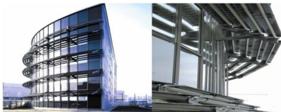
Fig. 3.B.29 SBL Offices Linz, Austria, Helmut Schimek, shading louvres with integrated photovoltaics and suntracking system, © Colt
